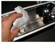
3. Obtain a napkin or towel free from debris, dirt, oil, etc. to remove the lamp with.
