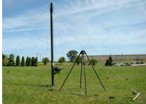
Figure 5-9 Position Gin Pole in Place with Its Center 3 Feet from Base of Mast
