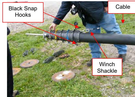
Figure 4-13 Connect Cable from Lift Winch to the Winch Shackle
