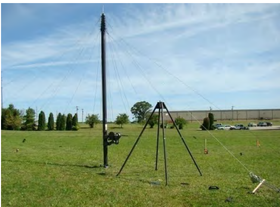
Figure 4-18 Raise Mast to Vertical
